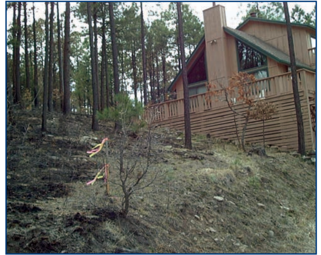
The pre-fire activities implemented by this homeowner include a maintained landscape, use of Firewise plant materials, reduced vegetation around the perimeter of the property and fire-resistant roofing material.
